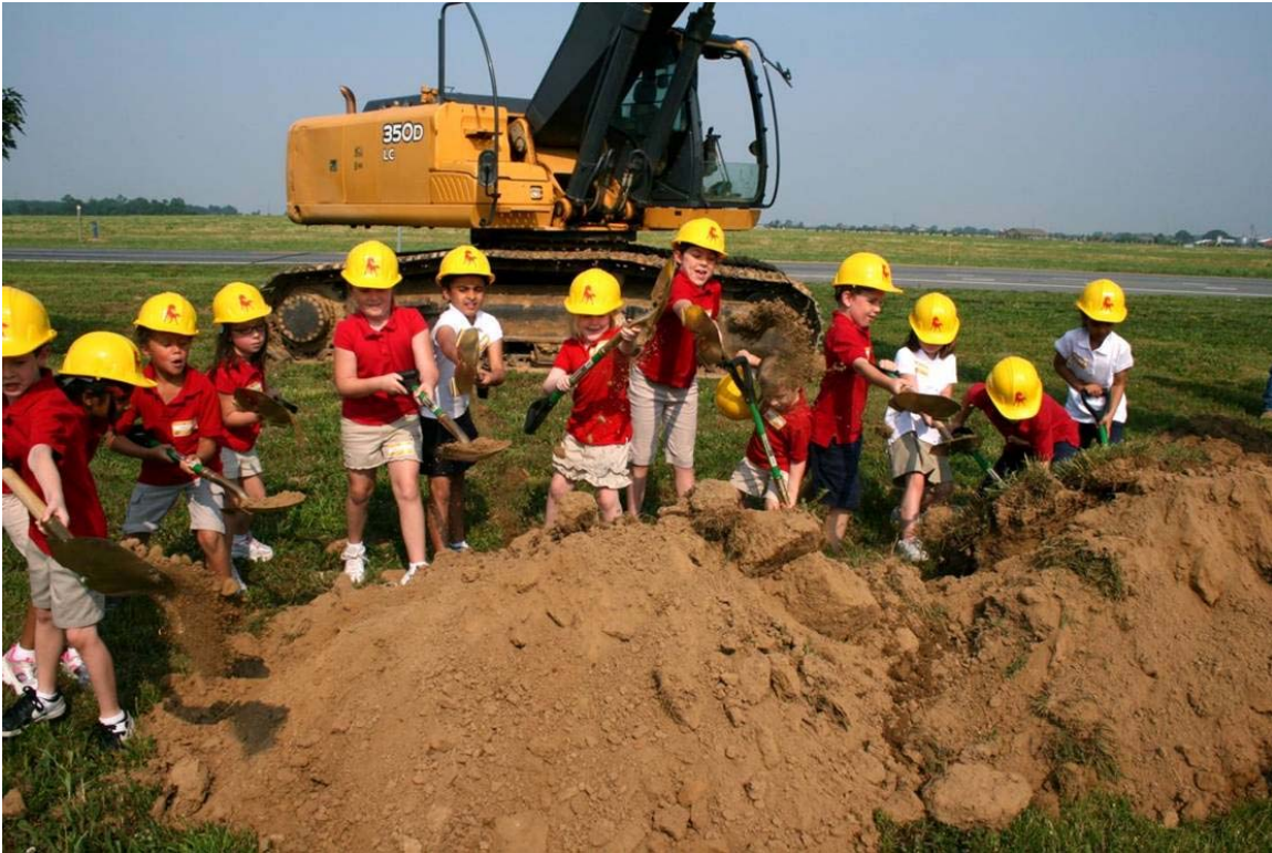
MOT Charter students help to break-ground for the new addition
